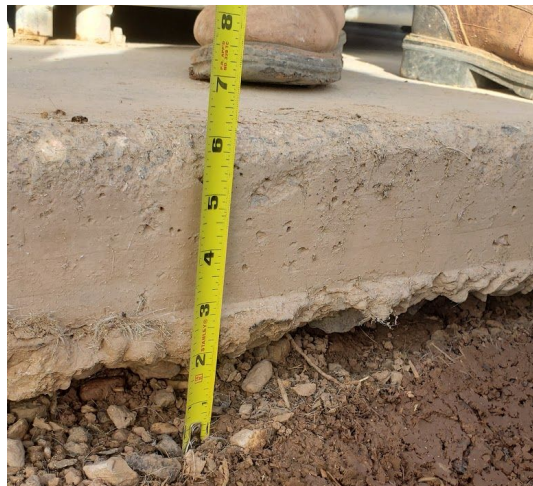
Figure 3-4: Measurement of the existing slab.
